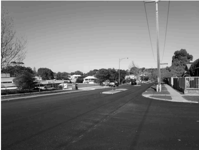
Monument Street – an avenue crying out for trees.
